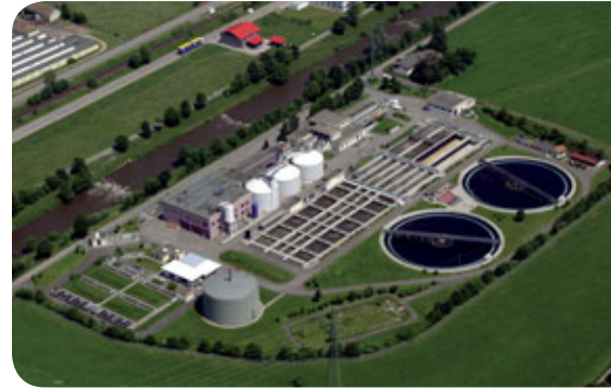
Steinen sewage treatment plant
