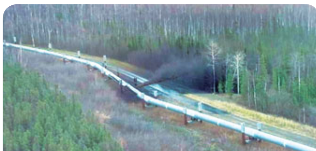
Image, left: leak in a pipeline. Image, right: contaminated/blocked pipeline.
