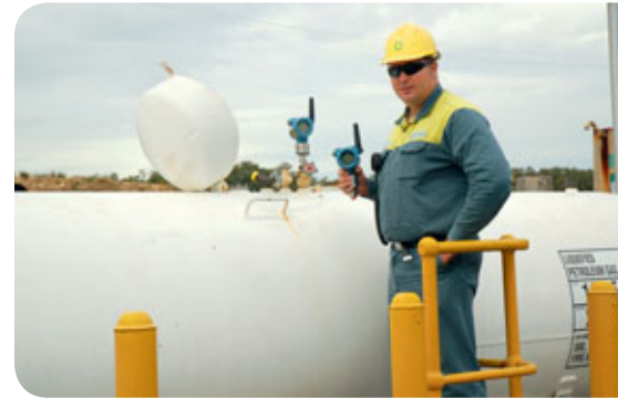
Mobile measurement with wireless pressure transmitter
