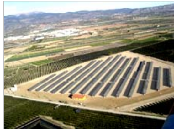
Totana PV solar plant, Spain
