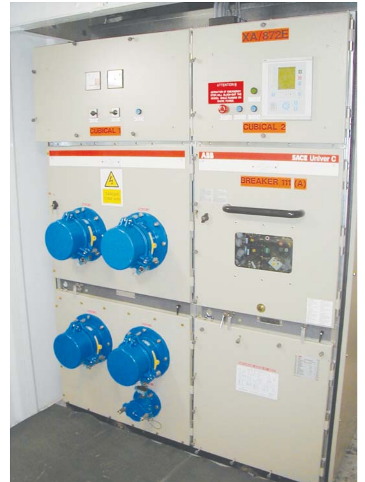
Figure 2 shows a ship with diesel machinery and low voltage electric system. The Shore Connection System is arranged with the Shore Connection Panel located outside the main switchboard room with cable connectors mounted in the front. An onboard transformer steps down the power from high to low voltage.
