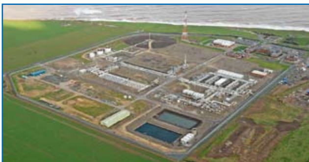
BP Dimlington Gas Terminal
