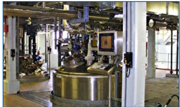
Inside the KemFine plant at Grangemouth
