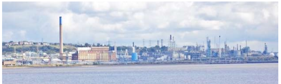
Existing INEOS ChlorVinyls site in Runcorn.
