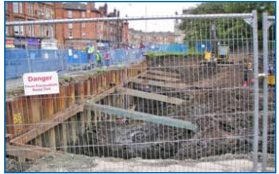
Ongoing demolition work
