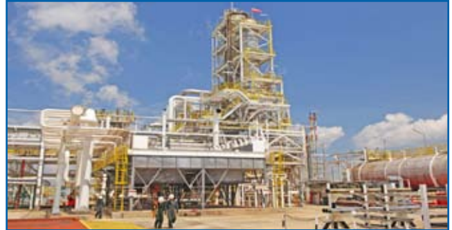
Petronas plant in Malaysia
